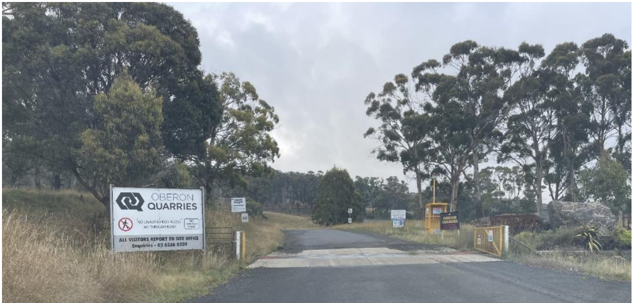
Quarry - Site Entry
