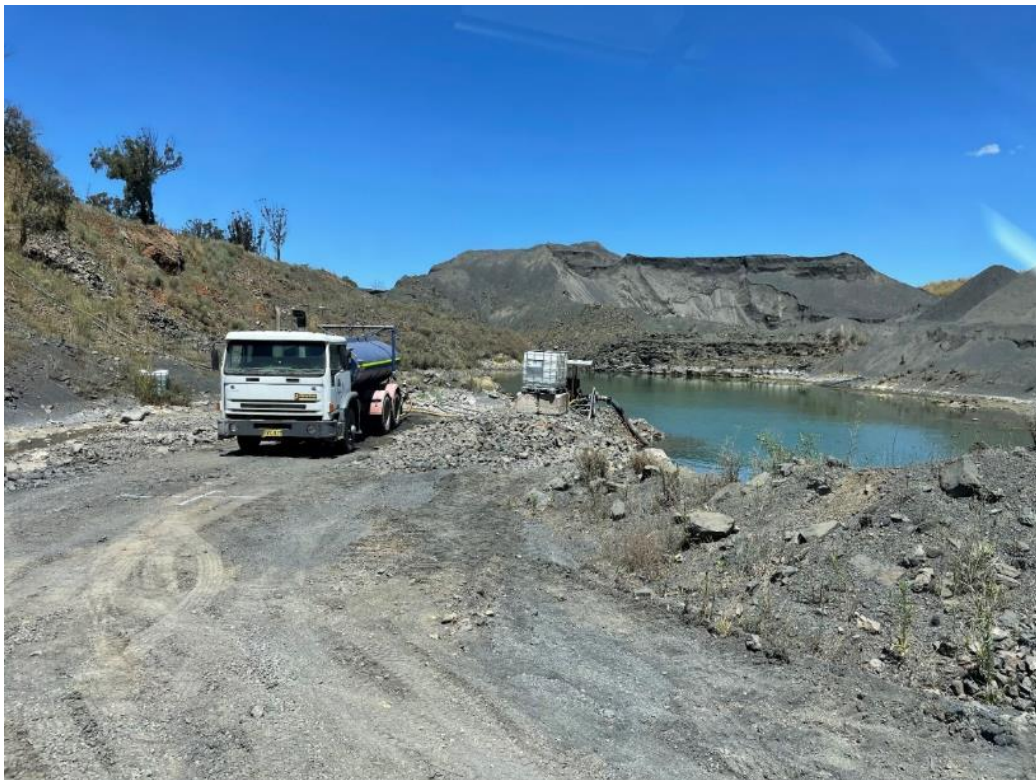
Quarry internal storage and Water Cart.
